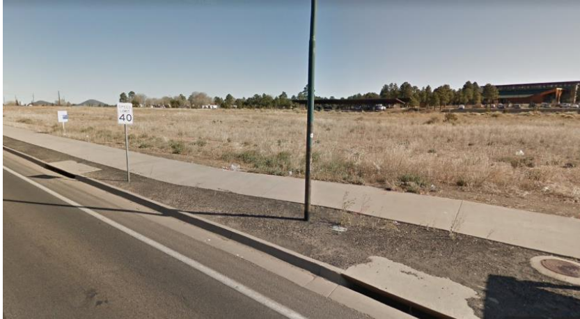
Figure 4-2: Catch basins along route 66
