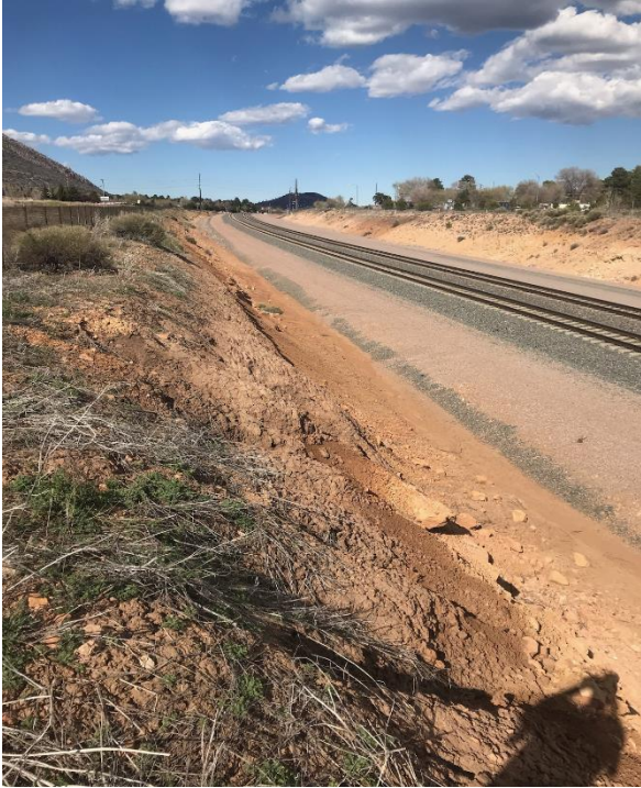
Figure 1-2: Back slope location facing east
